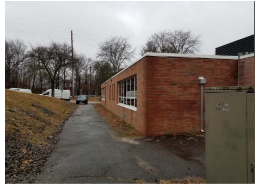
PHOTO A - Rear Drive New Gas Service From Central Ave To be Run Down Drive To Wall Adjacent To Transformer. Coordinate With Electrical Lines From Utility Pole To Transformer
